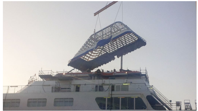
An exhaust gas cleaning system being fitted on our ships
